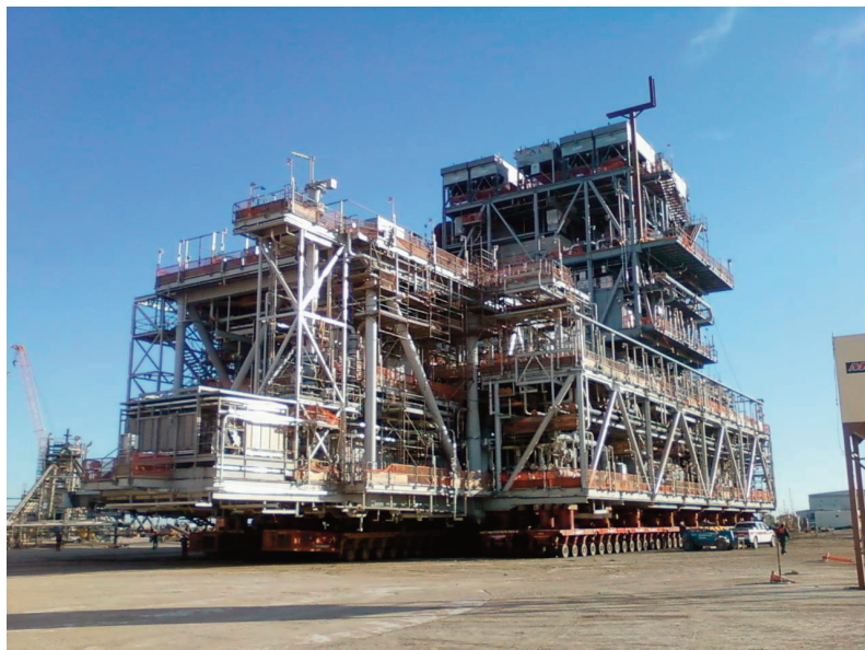
Process Module being moved to Transport Barge
