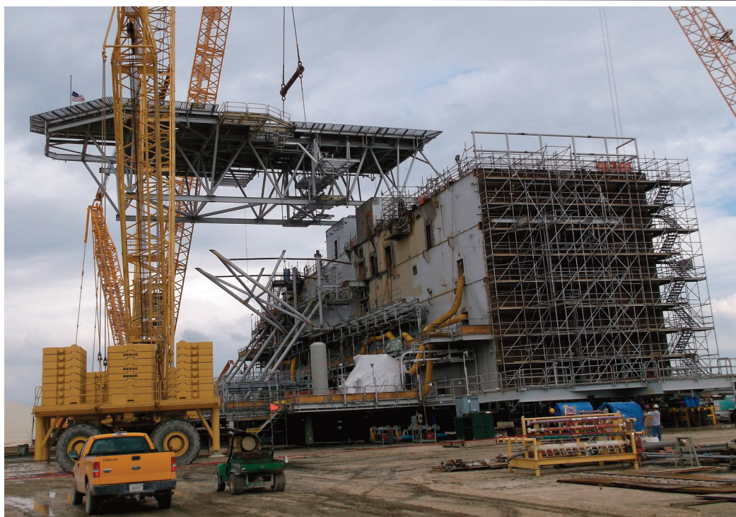
Helideck lifted onto the Quarters Module
