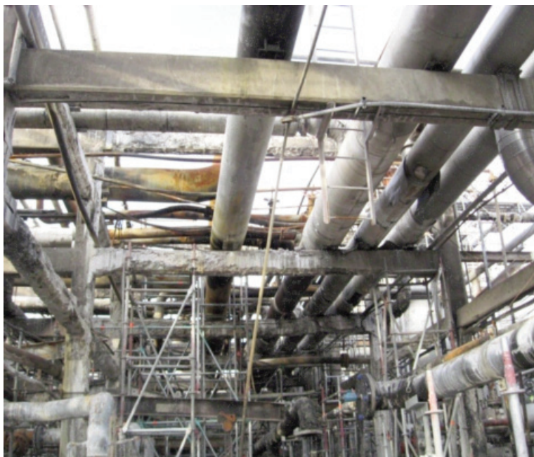
Close-up View of Original Concrete Piperack Bent
