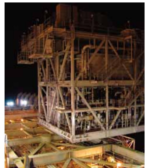
UPWF Project - 675 Ton Water Injection Module Setting
