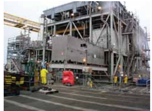
Crosby Gas Compressor Installation Project - Chemical Tank Skid Setting
