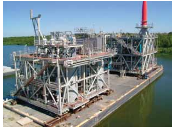
UPWF Project - Water Filtration Module and Sulfate Reduction Module Barge Transport
