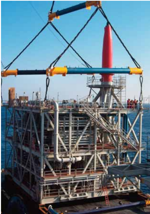
UPWF Project - 635 Ton Sulfate Reduction Module Lift
