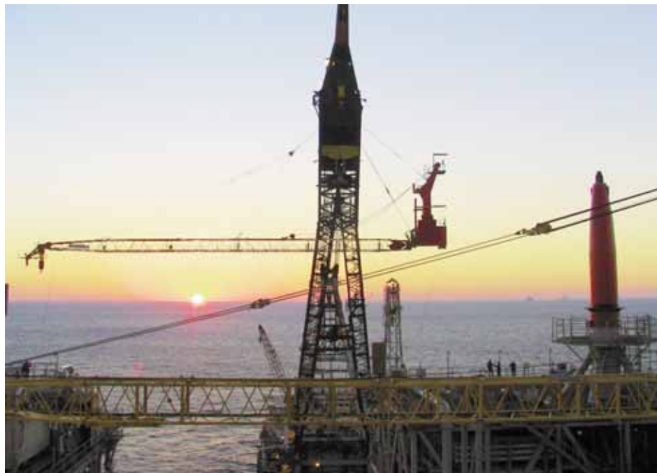
UPWF Project - Platform Crane Lift View from TLP
