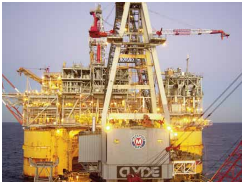
UPWF Project - Platform Crane Lift View from DB 50
