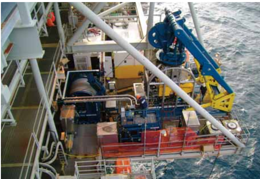
Temporary ROV Equipment Installation
