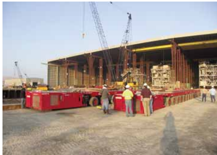
UPWF Project - Hydraulic Trailers used for Module Weighing and Loadout
