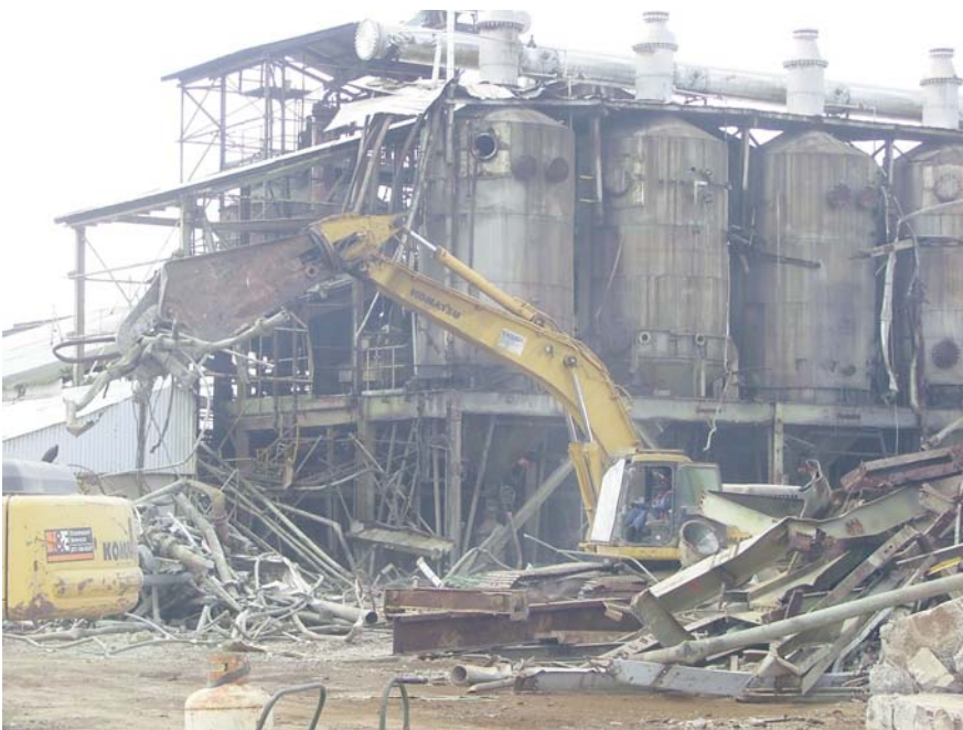
Structural demolition activities at an industrial facility
