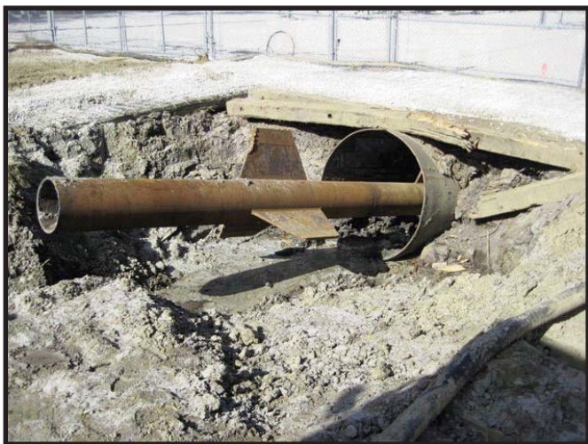
16-inch Centralizer Pipe in 60-inch Casing
