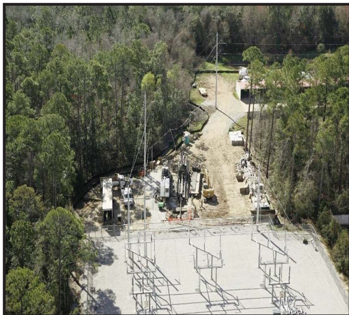
Florida Avenue Substation Directional Drill Rig
