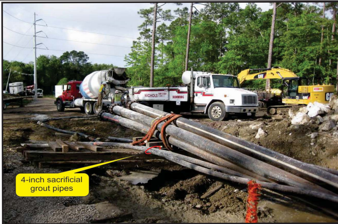
Thermal Grout Installation
