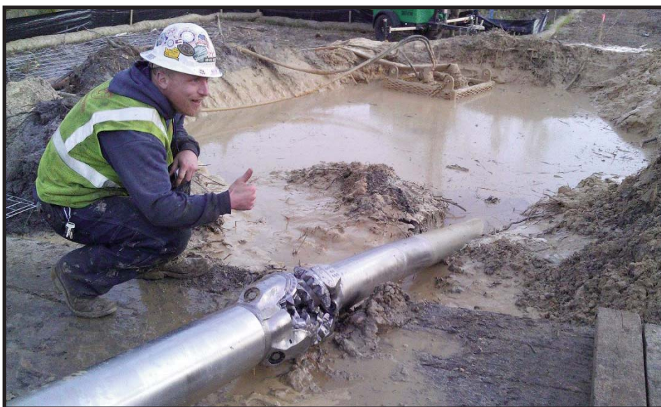
Sapling Point Exit of Both Drill Bits
