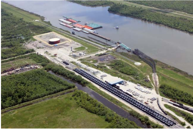
Innovative Rail to Barge Transfer Terminal Developed on Brownfield Industrial Site
