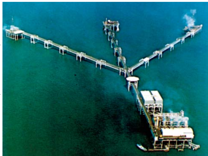
World Record Offshore Platform Complex Designed in 1957
