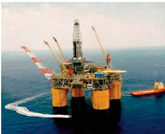
Tension Leg Platform For Oil & Gas Production
