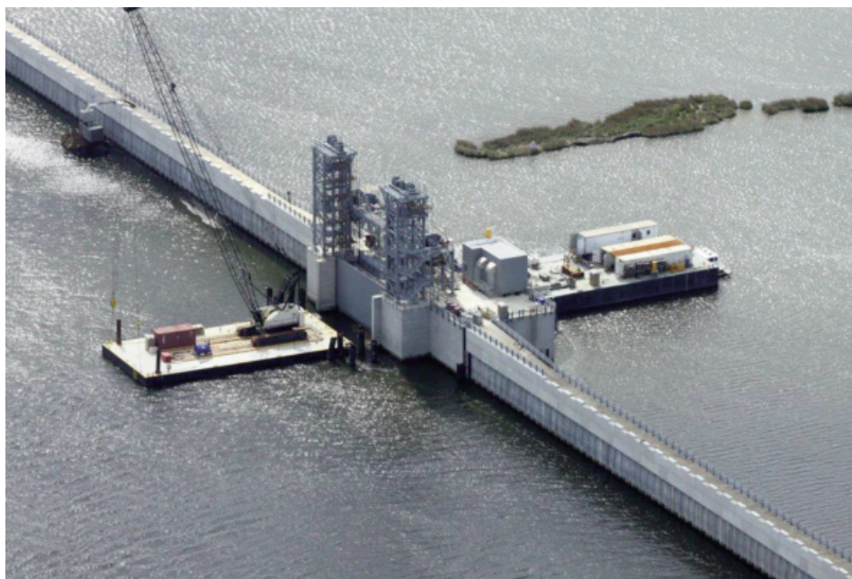
Photo during construction of the storm surge barrier east of New Orleans after hurricane Katrina. NELSON designed the lift gate for one of the navigation openings in this structure.
