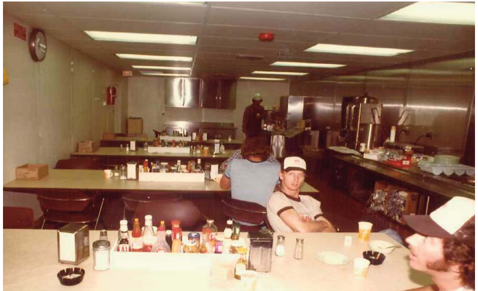
View of the galley when the Mr. Charlie was in operation
