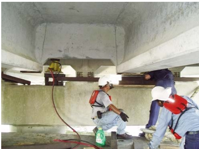
Fig. 4: Jacking Spans Back In Place (Photo Courtesy of Boh Bros.)
