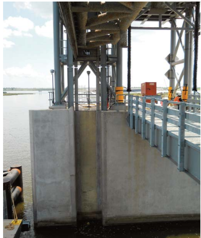
Lift Gate Slots and Access Bridge
