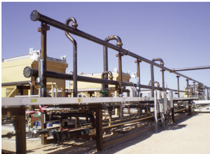
CPF facilities were designed with a modular concept including pipe racks to minimize field construction.
