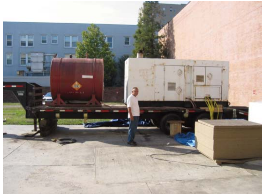
Hooking up temporary power for our building after Hurricane Katrina
