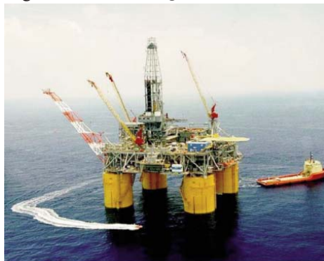
Remote operations such as offshore oil platforms require total self sufficiency in power generation
