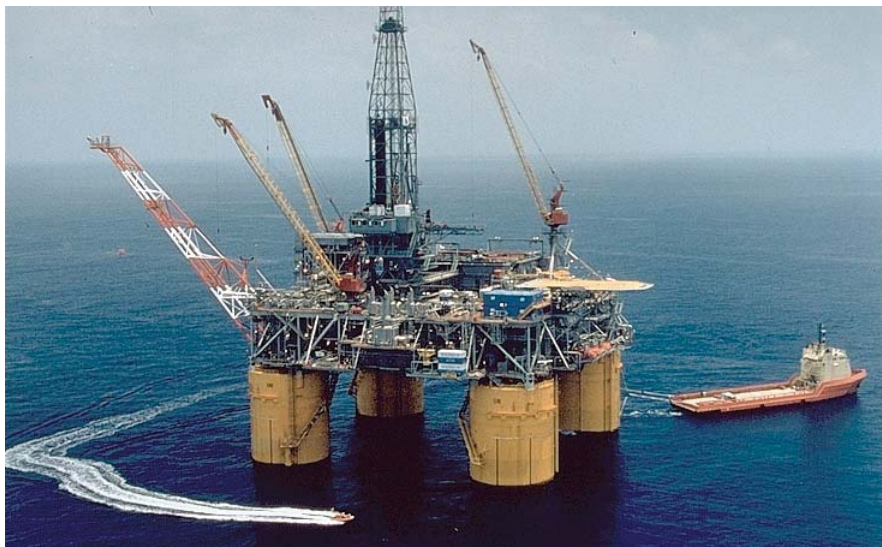
Tension Leg Platform Installed in Gulf of Mexico
