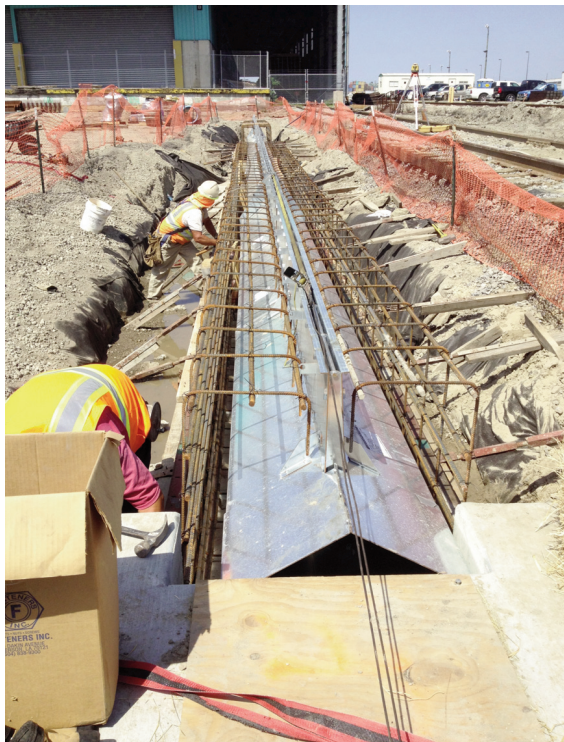
Slotted drain system ready for concreting
