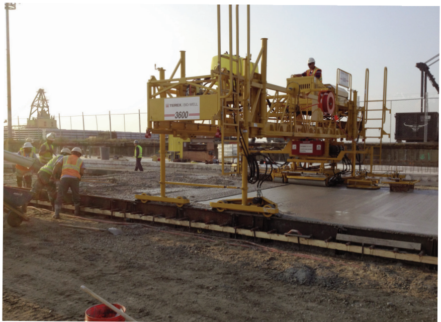
First paving sections being placed at Louisiana Avenue
