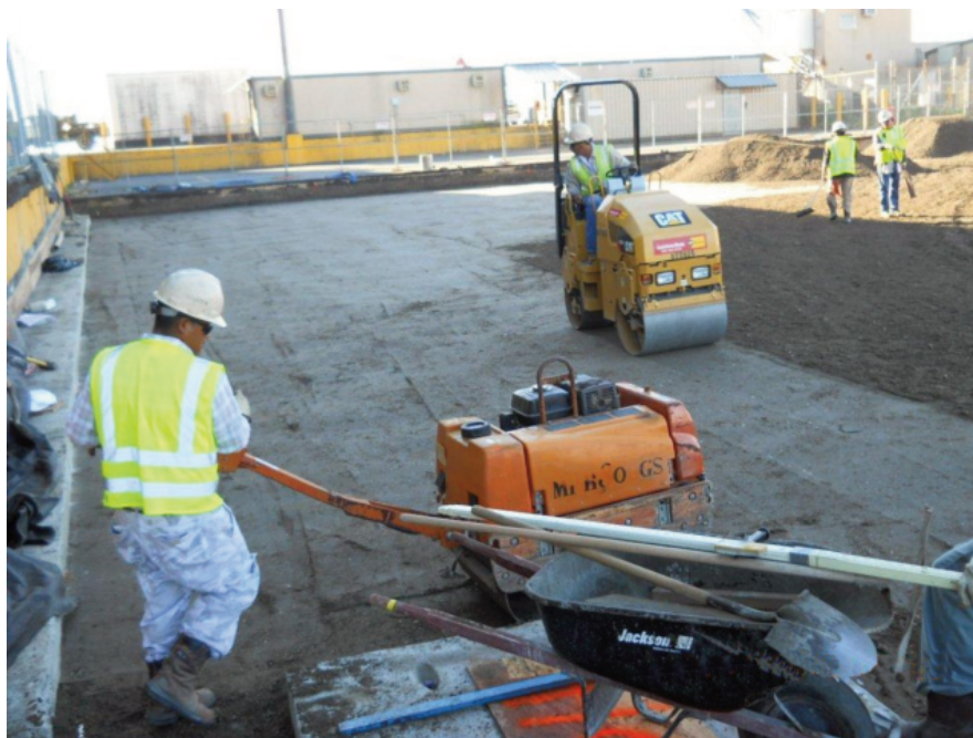
Pavement base undergoing compaction
