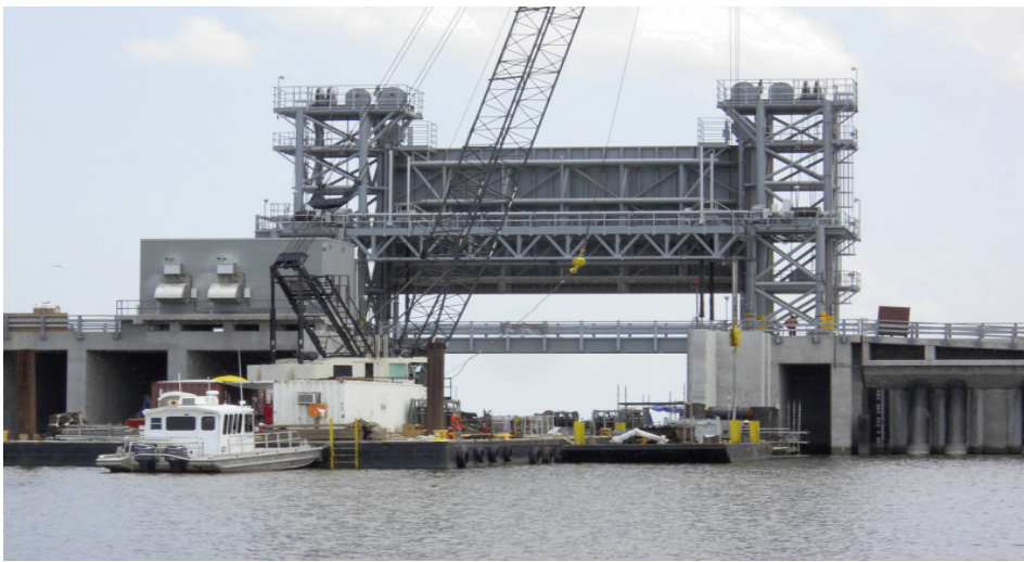
Bayou Bienvenue Lift Gate in the lifted position during construction
