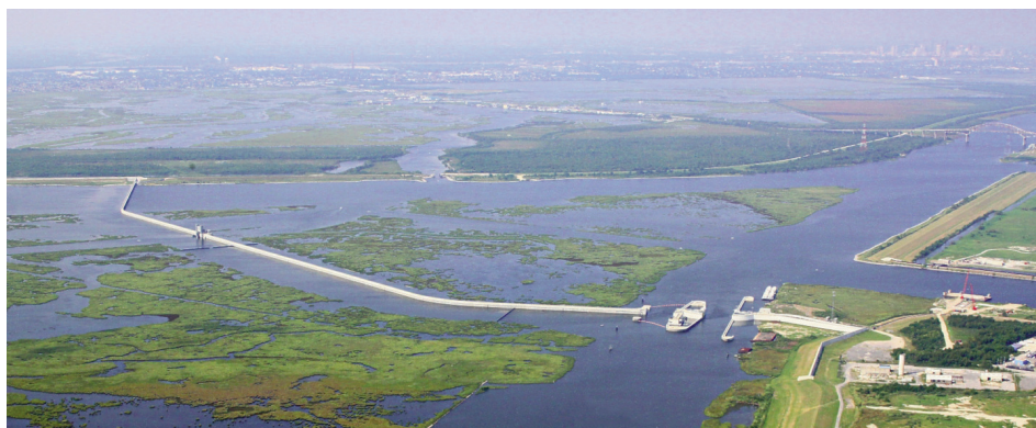
IHNC Surge Barrier extending from the MRGO on the left extending past the Bayou Bienvenue Lift Gate on to the GIWW Sector Gate on the right
