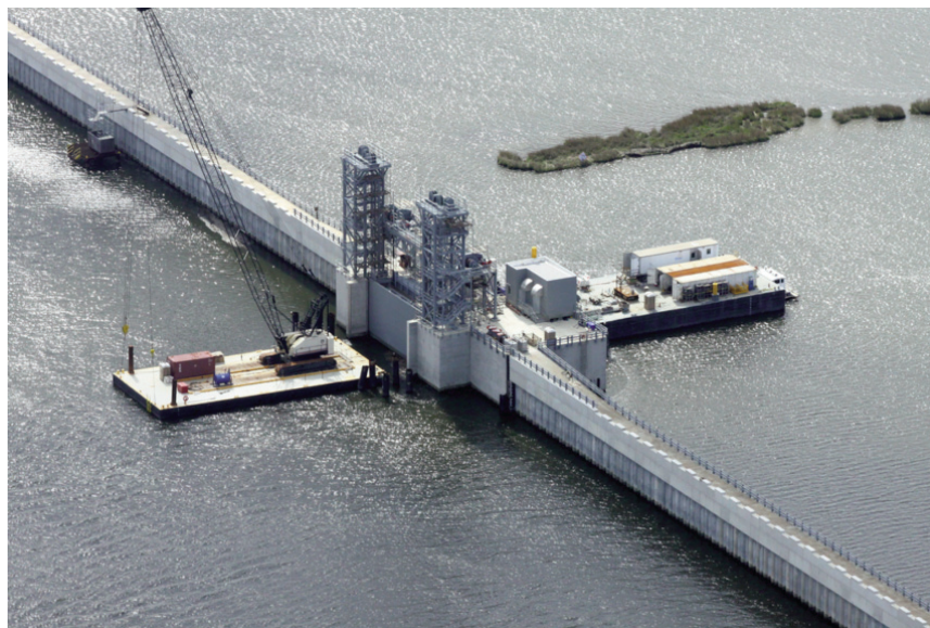
Bayou Bienvenue Lift Gate in the lowered position during construction
