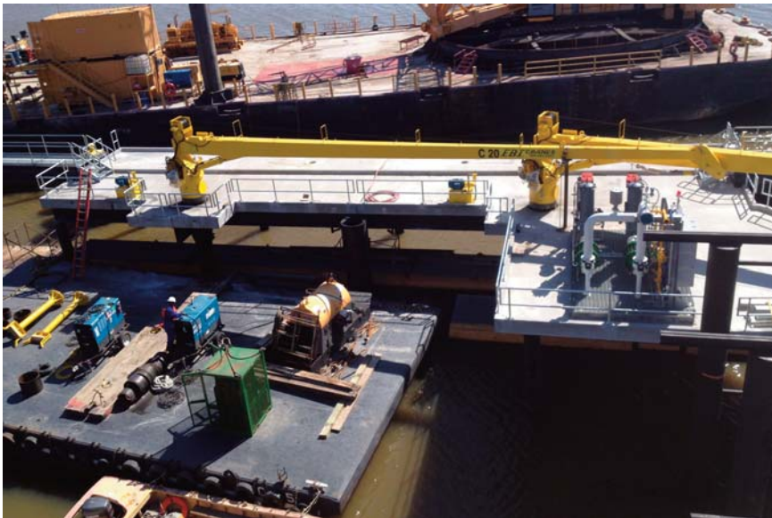
Marine Side Progress by Boh Bros. Construction Company
