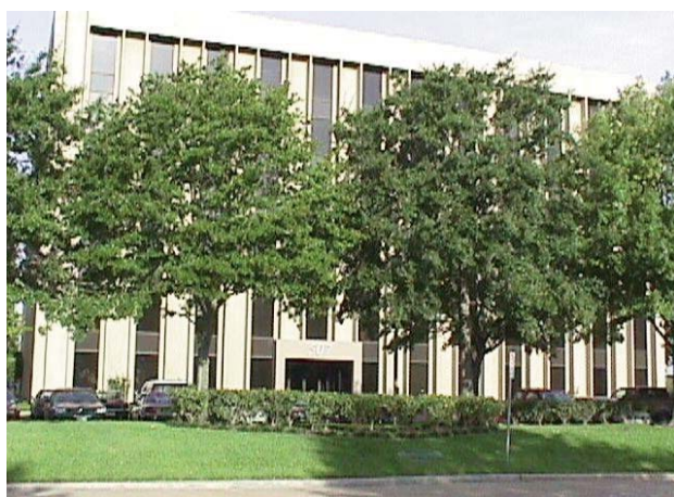
Sam Houston Parkway Building
