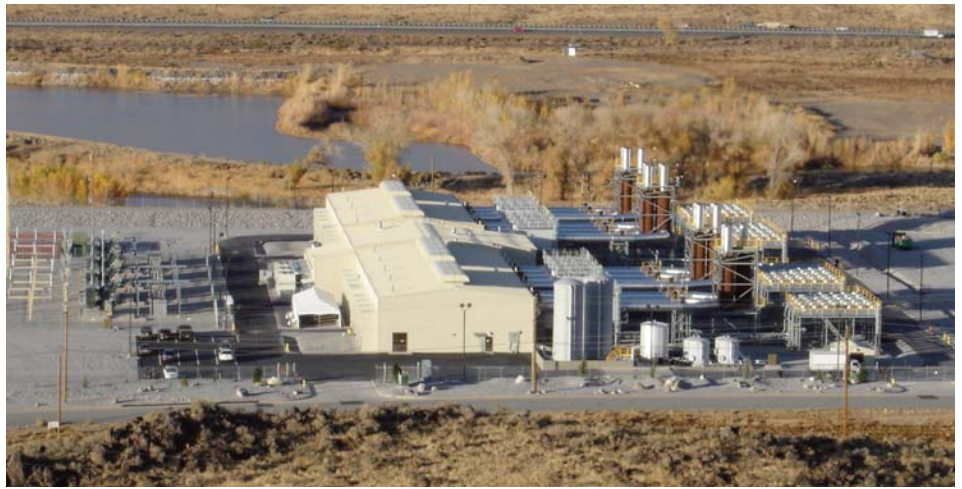
Wärtsilä Barrick Gold Mine Western 102 Power Plant
