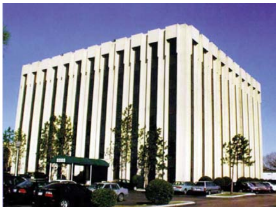
Voss Street Building
