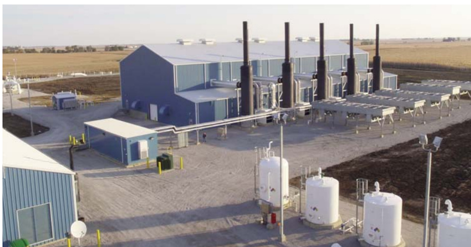
Typical Compressor Station
