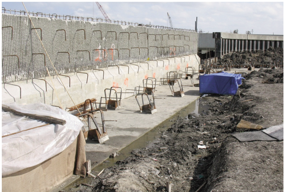
Preparation of existing I-Wall for bonding with new construction
