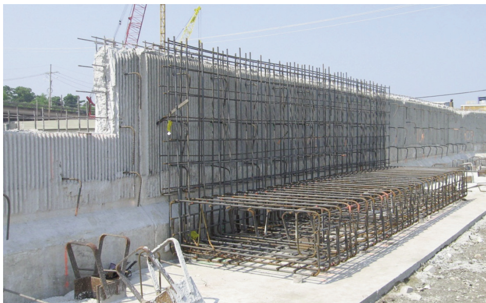
Construction of base and stem of floodwall
