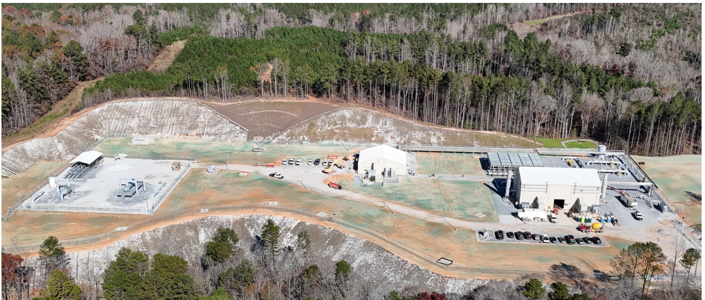
Rose Hill Compressor Station Southern Natural Gas Co.
