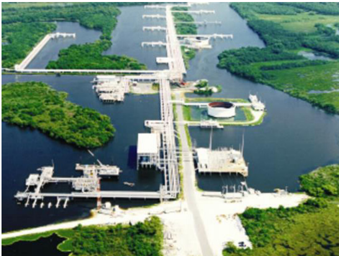
LOOP, Inc. Facility Expansion Shell Mars Project
